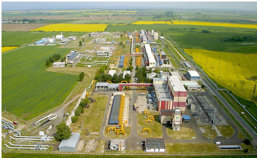
FIGURE 4: Largest EU compressor station in Slovakia [5]
