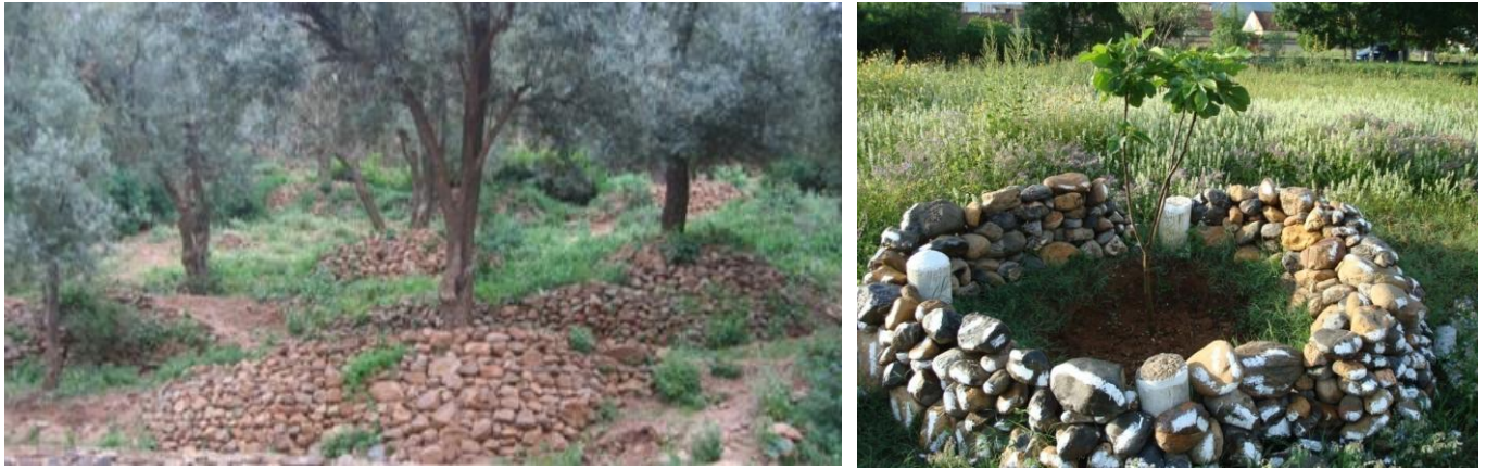
FIGURE 2. BASINS STRENGTHENED IN DRY STONES (BENI SNOUS AND BÉJAIA)
