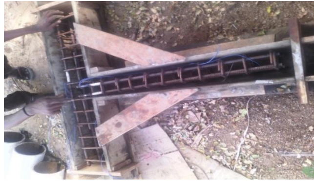
FIG.2 BEAM COLUMN JOINT MOULD
