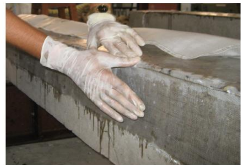
FIG 5 FIXING OF GFRP SHEET ON THE BEAM
