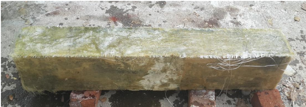
FIG 10 GFRP WRAPPING ON THE BEAM
