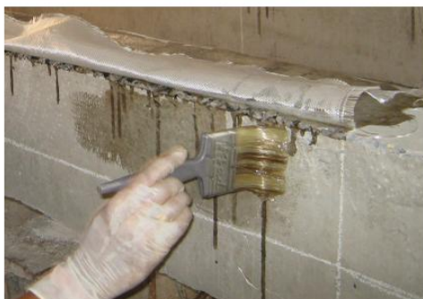
FIG 4 APPLICATION OF EPOXY AND HARDENER ON THE BEAM
