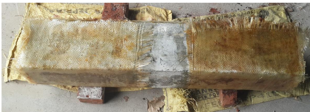
FIG 11 BINDING OF WOVEN MAT OVER THE GFRP SHEETS
