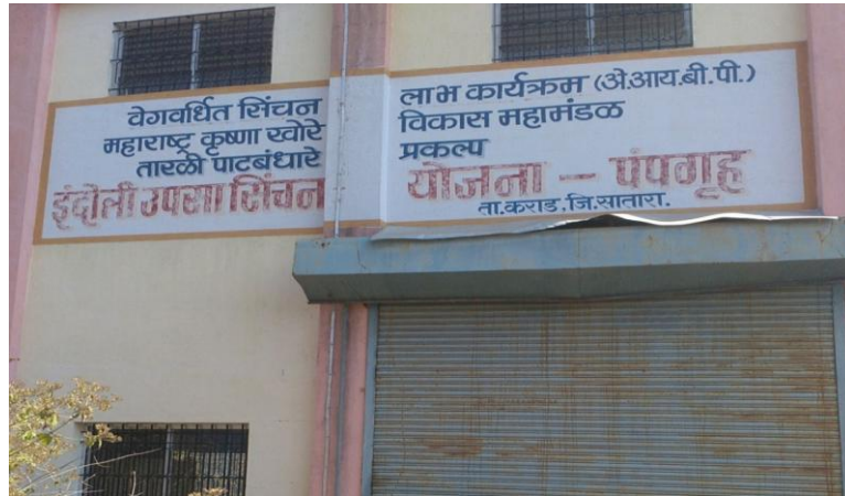
FIG 3.1 PUMP HOUSE AT INDOLI
